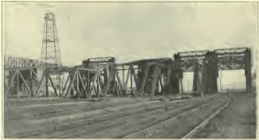
FIG. 270. BRIDGES. Rolling lift bridges over the ship canal at Indiana Harbor, carrying the tracks of the Chicago, Indiana & Southern Railroad, the Lake Shore & Michigan Southern Railway, the Baltimore & Ohio Railroad and the Elgin, Joliet & Eastern Railway.
